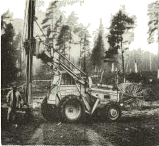
Fig. 2. Installation of drains
