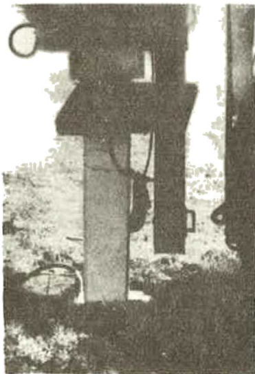
Fig.1.-Pile Driving in Polymer Jacket
