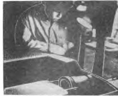
Fig. 9. Centrifugal model test of self-weight consolidation (in operation).
