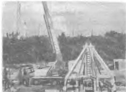
FIG.3. Loading frame of Fa. Frankipfahl
