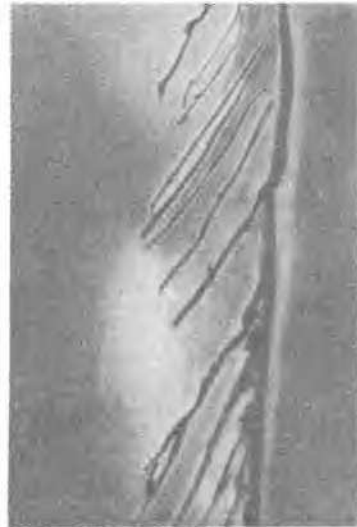
FIG. 3. PHOTO OF THE TRACES OF SHEAR EXPOSED BY CUTTING A HOLE
