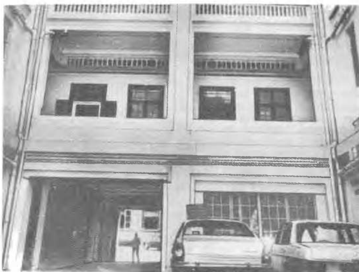
Figure 5 Crack patterns on beams
