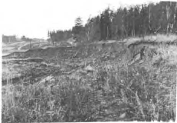
Fig. 6 Photograph Showing the Upper Part of the Failure
