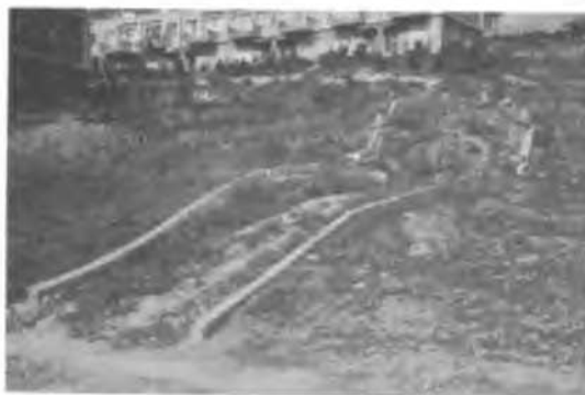
Fig.9 Destroyed road (R) on the sliding mass. See Figs. 1 and 3.
