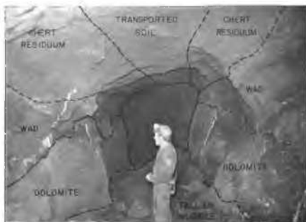
FIG. 4. An underground void of the type liable to cause a sinkhole.
