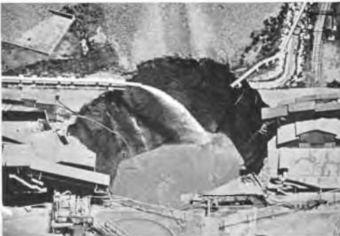
FIG. 1. Collapse of crushing plant into a sinkhole, Westdriefontein Mine, December, 1962. (Courtesy of the Johannesburg Star.)
