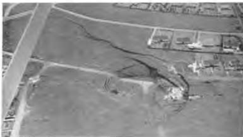
FIG. 2. A slow, caving subsidence of about 20-ft depth.
