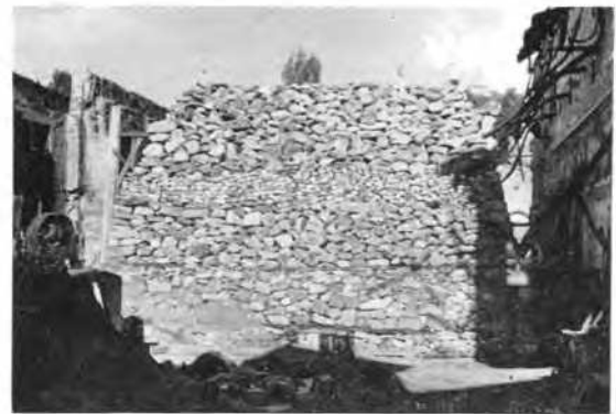
FIG. 9. View of the test loading arrangement.
