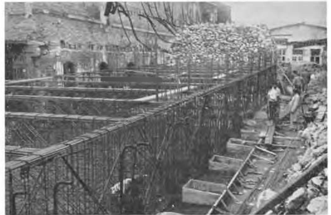
FIG. 12. Reinforcement of the box and injection tubes.
