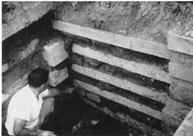
FIG. 8. Photo of crack illustrated by Fig. 9 (taken from opposite direction).
