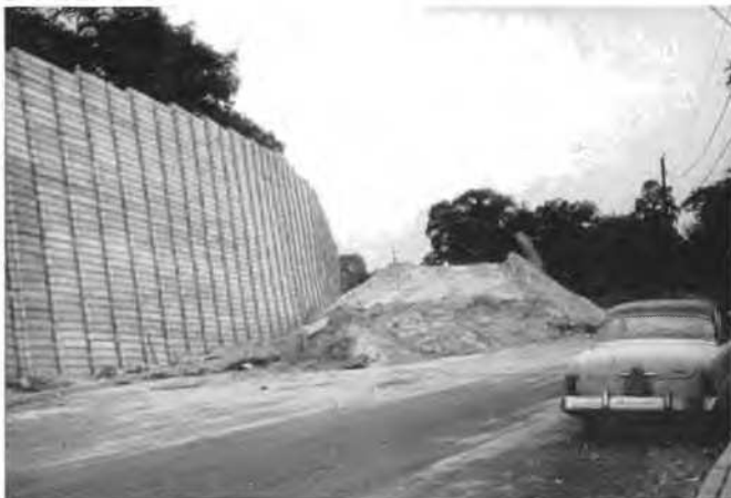
FIG. 1. General view of 34-ft high concave crib wall.
