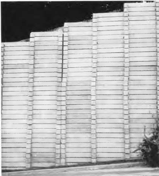
FIG. 4. Opening of upper part of expansion joint.
