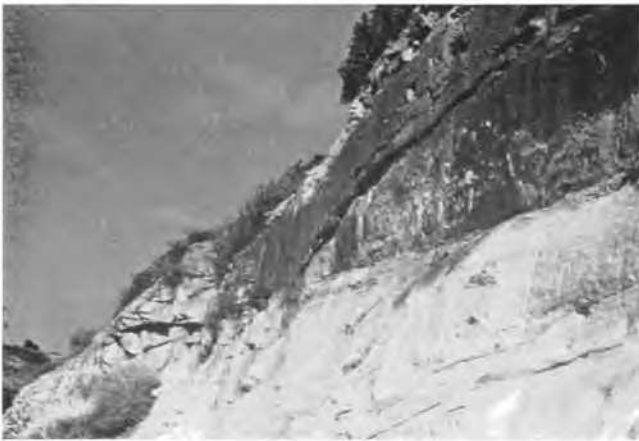
FIG. 2. Deconsolidation fissure cutting chalky cliff.
