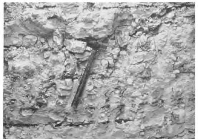
FIG. 6. Deconsolidation fissure cutting bedding in flinty chalk, at a depth of 2 m in test pit.
