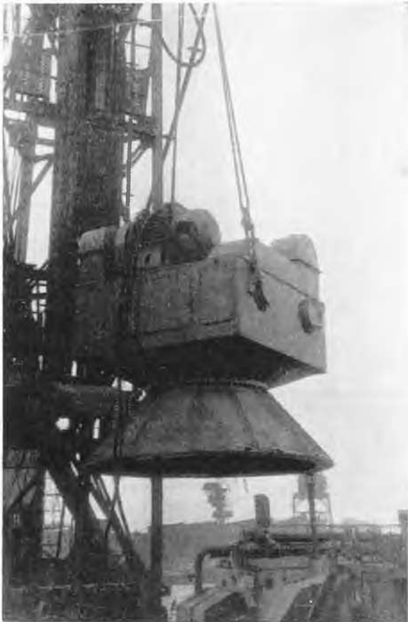
Fig. 1 The vibrator unit NVP-56 (designed by B. P. Tatarnikov).
