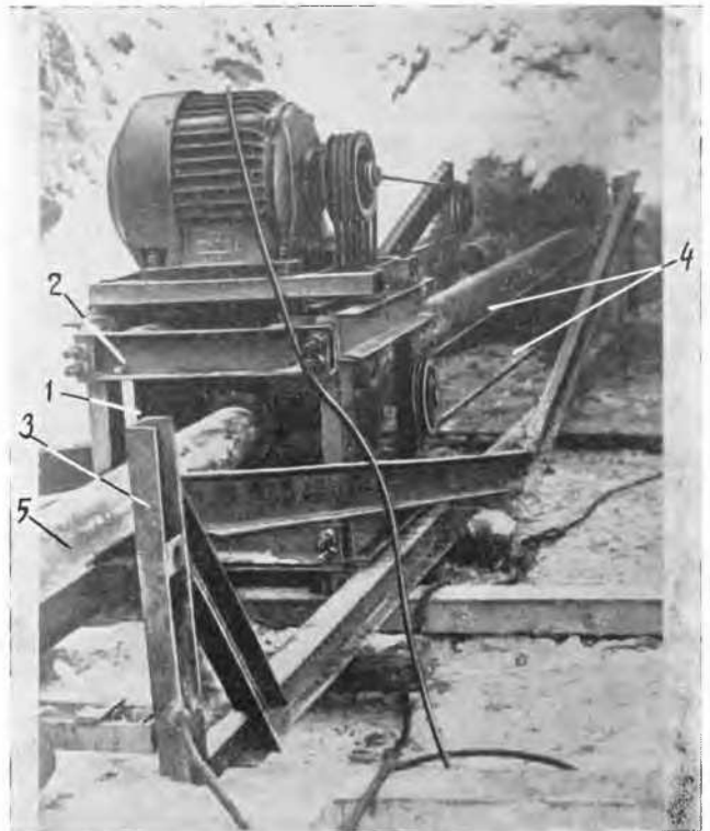
Fig. 2 The vibrator unit for laying pipes (designed by A. Ja. Luskin).
