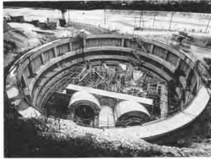
Fig. 6 Quero power station. Elliptical diaphragm. Usine de Quero. Mur diaphragme elliptique.
