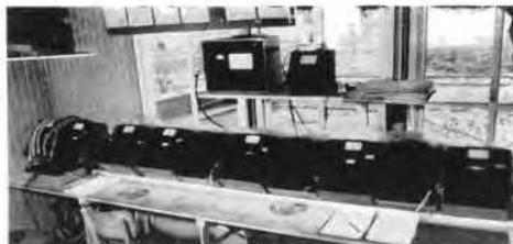
Fig. 4 Disposition of strain reading instruments in the shed.
