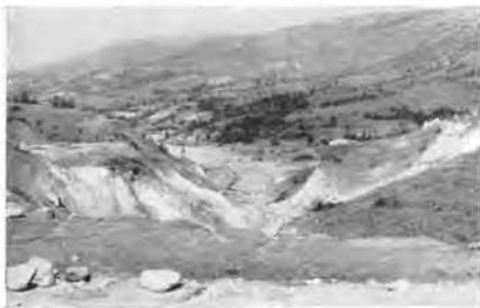
Fig. 3 The erosion bed created by the overflow of floodwater in 1957.
