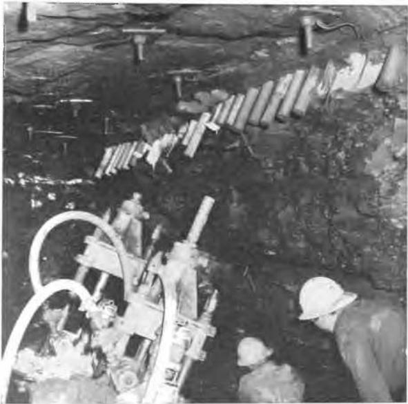
Fig. 34 Drilling stress relieving slots and insertion of wooden dowels.
