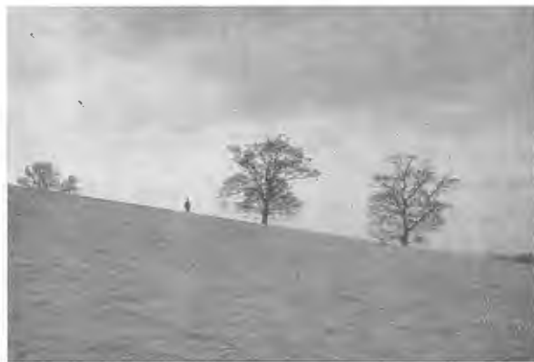
Fig. 5. Sewardstone No. 5. 10 degree slope, stable Talus à 10 degrés, stable
