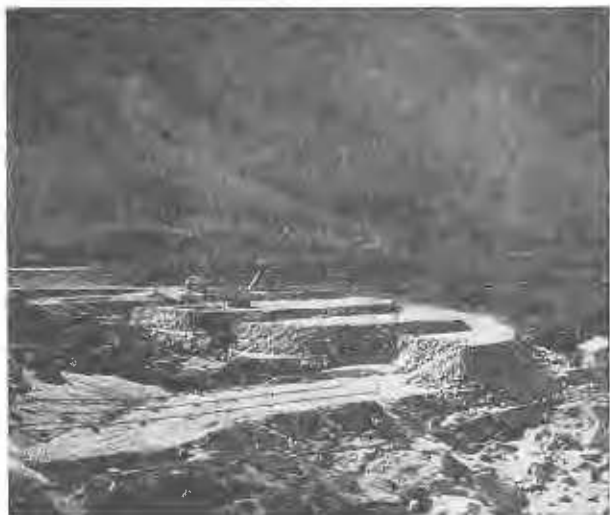
Fig. 4 General view of test fills. Foreground: sluicing operation. Middle ground: excavation of test pit for density determination
