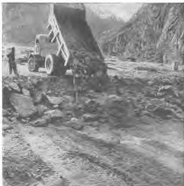
Fig. 6 Test fill No. 2: dumping of wet material right on the edge of fill to reduce rolling distance (2.0 m lift)
