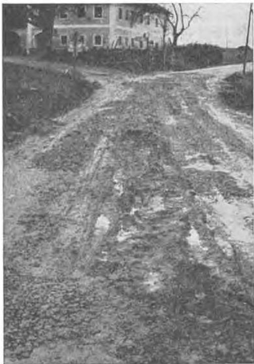
Fig. 19 Before stabilization the road showed heavy frost damage after every winter
