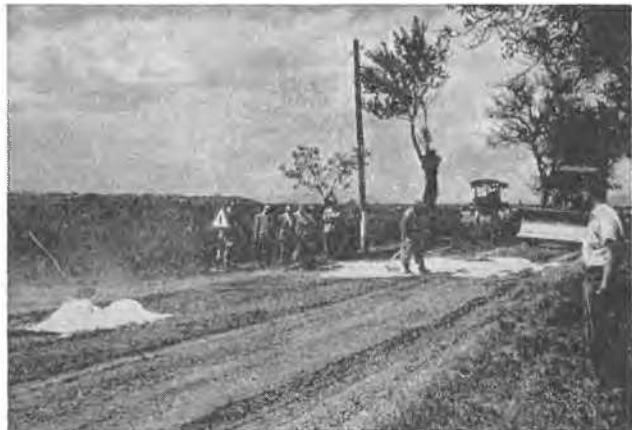
Fig. 20 Applying hydrated lime by hand
