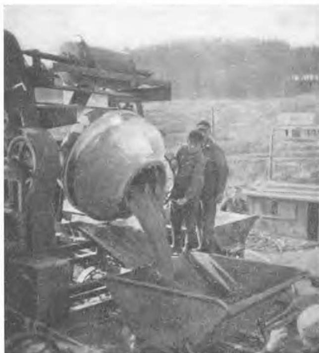
Fig. 2 Discharge of the Prepared Limit Mix from the Gravity Mixer (Type Jäger)
