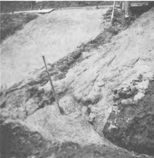
Fig. 6 Discharge of the Mass on a 1 : 2.5 Slope and Filling of a Ditch. While the Mass Still Flows Down the Spade Stands in the Thixotropically Cohesive Mass
