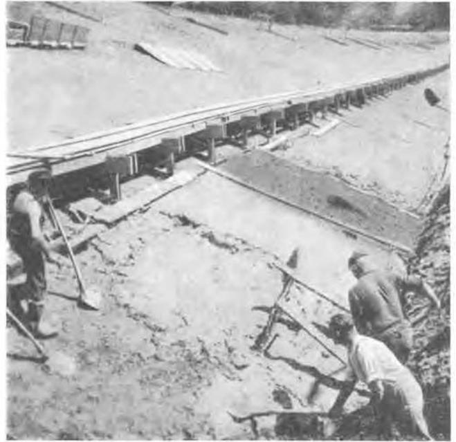
Fig. 10 Survey of the Application of a Chemical Carpet at the "Cranzahl" Dam in Strips of 3–4 m; Left Above the Transport Bridge; in the Foreground Placing Work, at the Back: Finished Chemical Carpet
