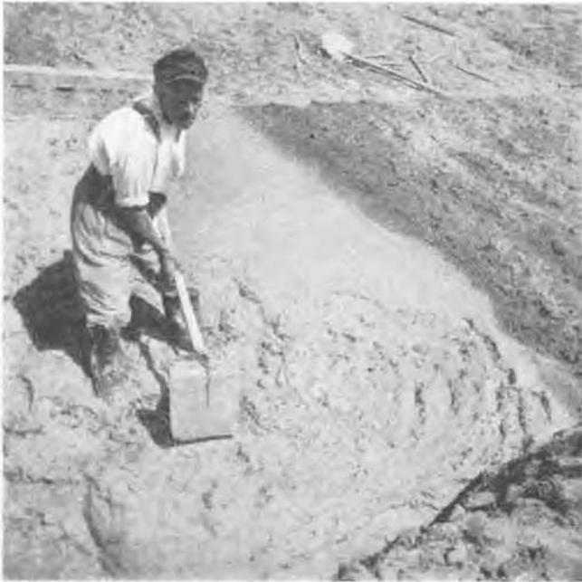
Fig. 9 Application of the Material by Hand—Left Foreground. Right: Freshly Finished Chemical Carpet as a Protection Against Drying-up
