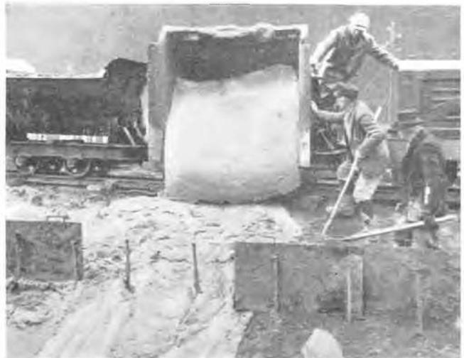
Fig. 4 The Thixotropically Cohesive Mass is Discharged as a Whole
