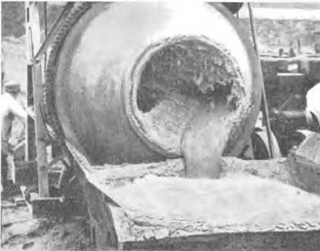
Fig. 3 Discharge of the Viscous-Pulpy Mix from the Forced Mixer (Type Kaiser)
