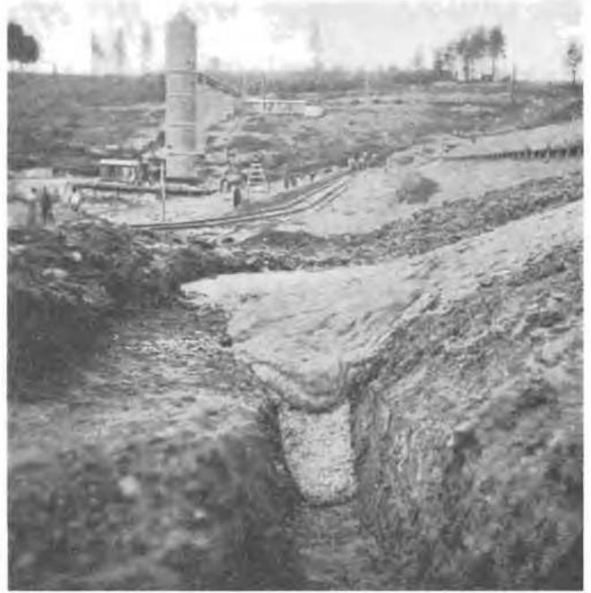
Fig. 7 Filling of the Ditch on the Water-Side Base of the Slope of the "Cranzahl" Dam (Saxony)
