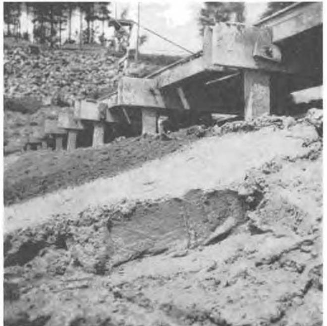
Fig. 8 Application of a "Chemical Carpet" of a Thickness of 20 cm on the Water-Side, Slope 1 : 3 at the "Cranzahl" Dam. The Stabilized Mass Stands Vertically Like a Stiff-Plastic Loam
