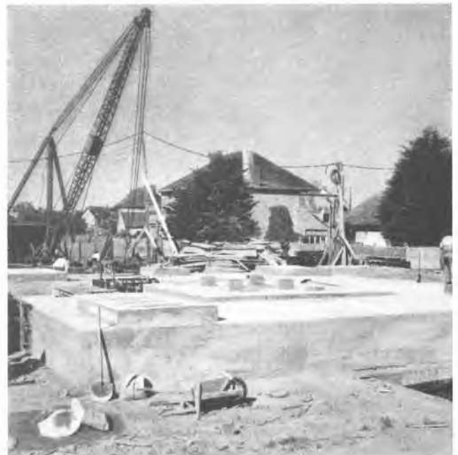
Fig. 9 Travaux terminés Completed Work
