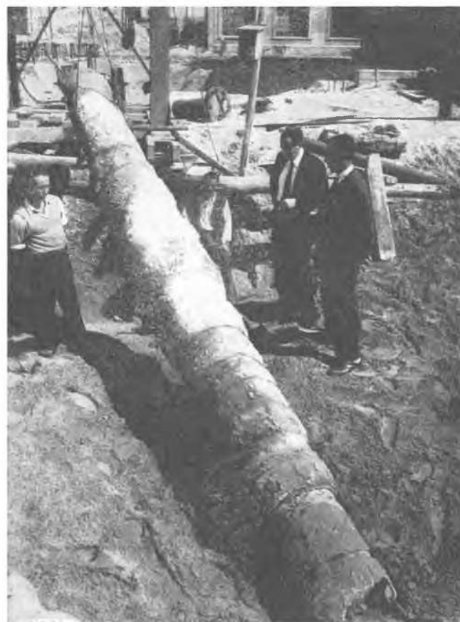
Fig. 5 Pieu arraché Uprooted Pile
