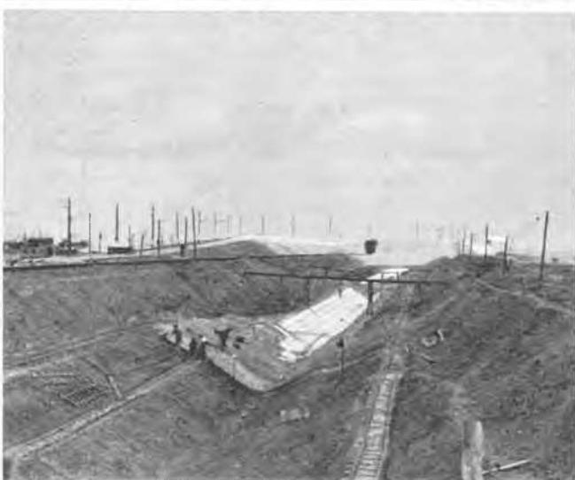
Figs. 11/12 Hydratop Stabilizing Carpet on the Loam Banks—Slope 1:1.7—of a Drainage Ditch in the Brown Coal District of Central Germany. Loess Loam: Liquid Limit 25%, Water Content 38%
