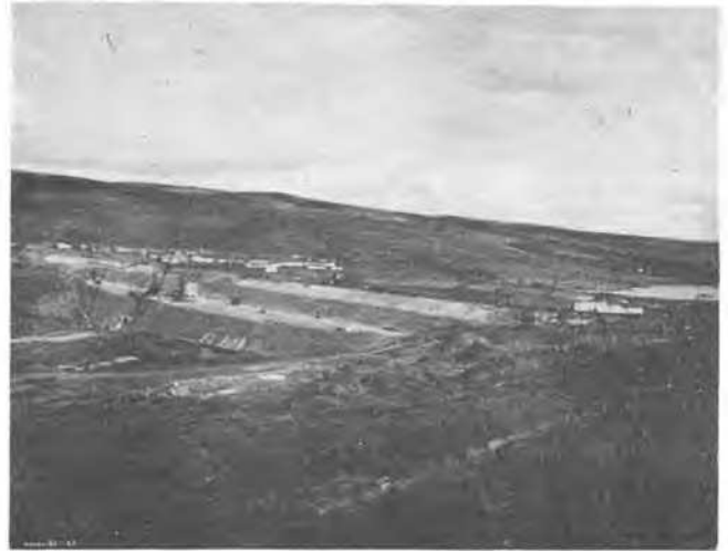
Muirhead reservoir. Upstream face of dam.
