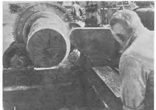
Pile-turning machine. Close view.
