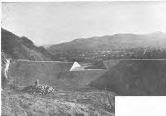
Upstream view of completed structure.
