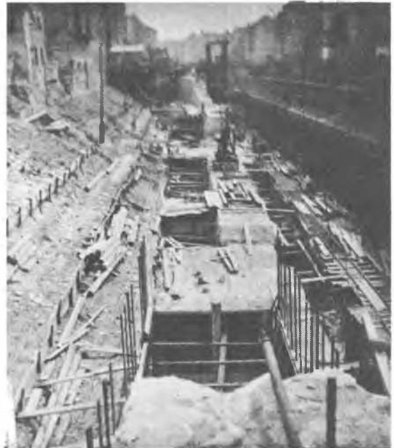
Downstream view of stage of repairwork on 2 nd July 1947.
