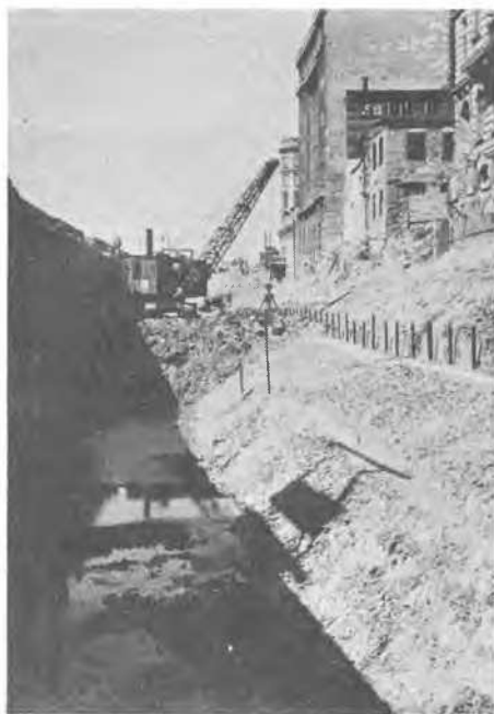
View of excavation behind the displaced wall, taken upstream from bottom of the trench on 3rd August 1946.
