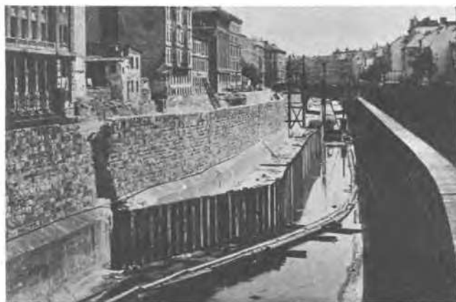
Downstream view of sheetpiling, taken on 3rd August 1946.
