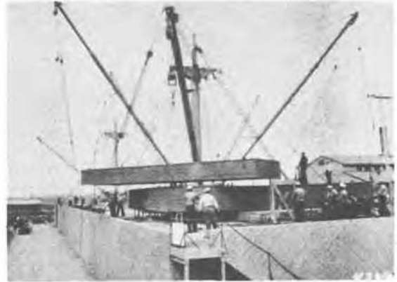
"Jumbo" boom in operation handling LCM and LCVP boat mockups.
