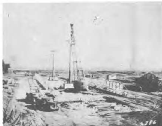
The second mast is lifted and placed on base. FIG. 3
