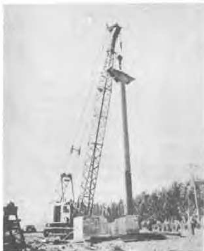
Crane placing mast on concrete foundation. FIG. 1
