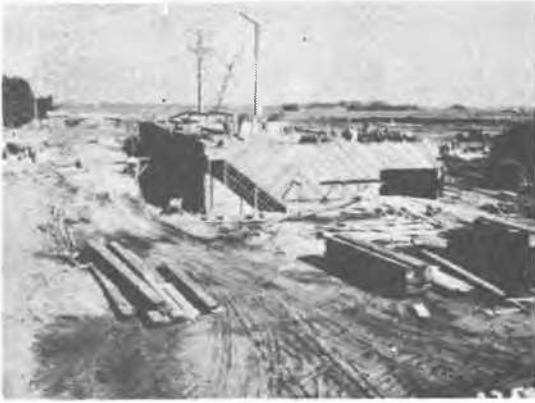
Construction of Stevedore Training Ship in progress.
