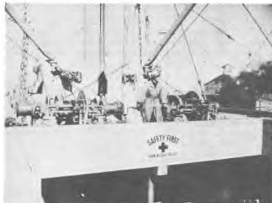
Completed pedestal with booms and gear. Operation of winches. Boiler house at right.
