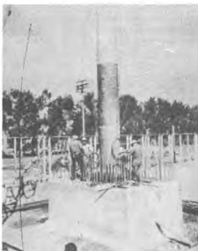
Close-up view of mast on concrete foundation. FIG. 2
