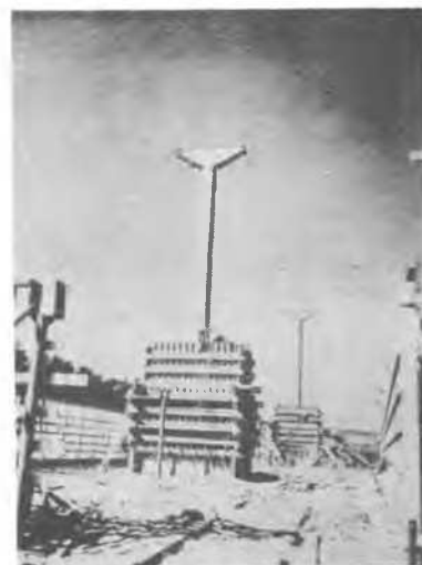
Forms for concrete pedestals. FIG. 4
