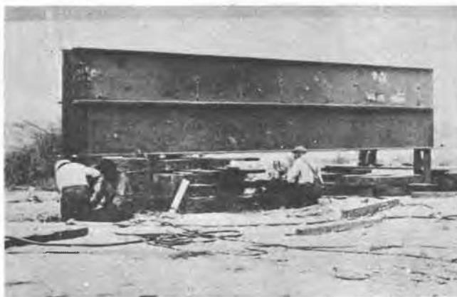
Assembling 200-ton-capacity reaction frame.
