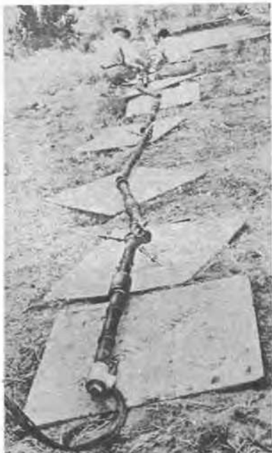
Assembling 5-foot sections of pipe preparatory to installing in pile.
