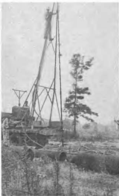
Installing assembled unit in pile.
