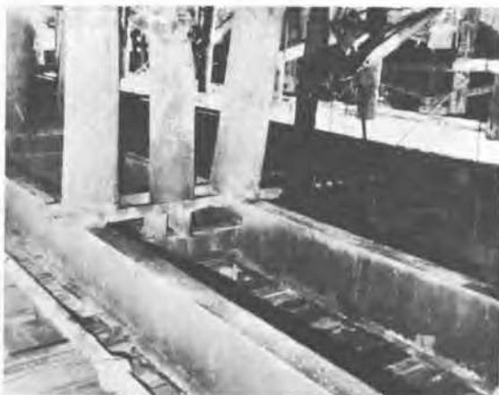
Condition of old wharf in September 1941.
