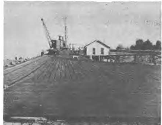
Reconstructed wharf showing locomotive crane and Mississippi River levee.
