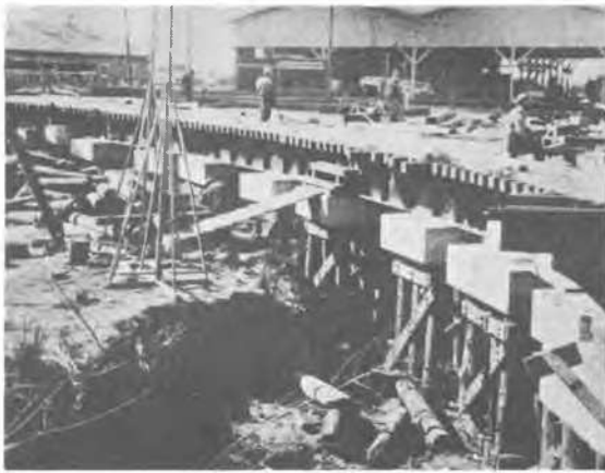
Curved approach to wharf showing concrete caps on pile clusters.
