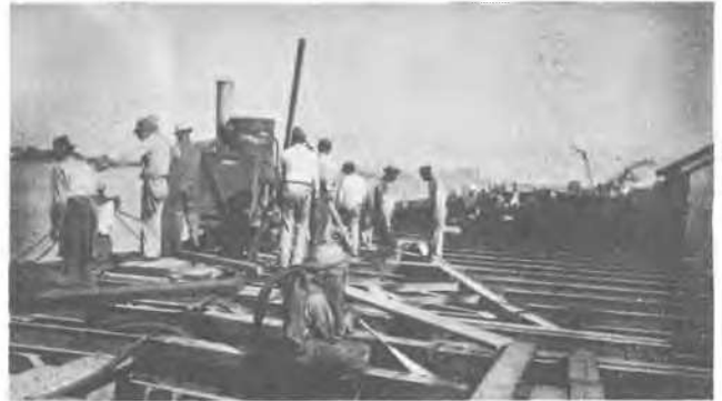
Sand blasting, cleaning, and painting steel beams on wharf.
