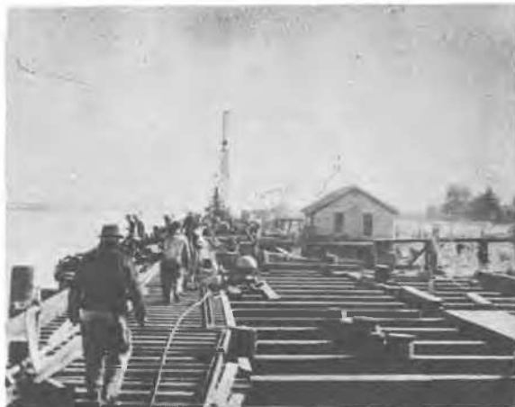
Looking east - wharf reconstruction - laying railroad rails.
