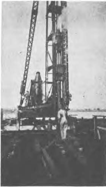
Pile driving operations on wharf.
