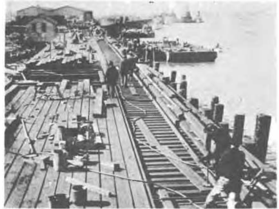
Facing west - construction of timber decking and railroad track.
