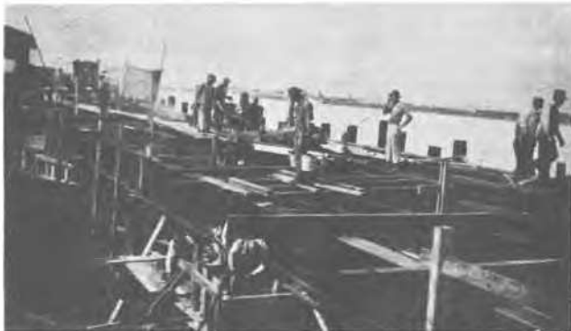
Building forms for concrete caps for wharf.
