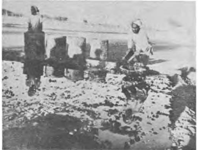
Pouring water for optimum moisture over a wearing course stack.
