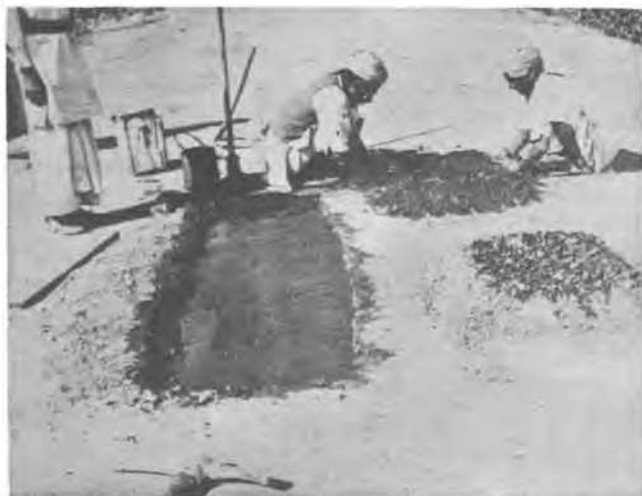
Patch repairs.
