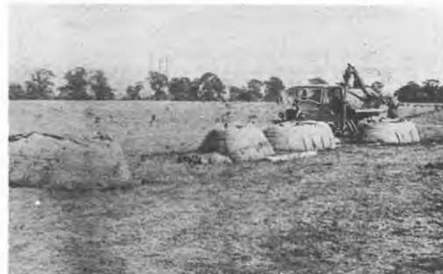
Gully - emptier shown filling canvas water dams.
