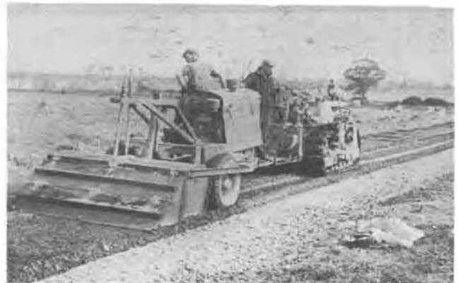
"Seamans" Motorised "Pulvimixer" rotary soil-mixer. (Mixing water into six foot width of soil cement).
