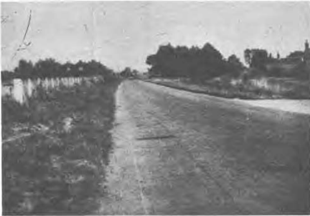
Abingdon:- Part of the soil-cement section as it was in 1947. (N.B. The marks on the road are caused by oil).
