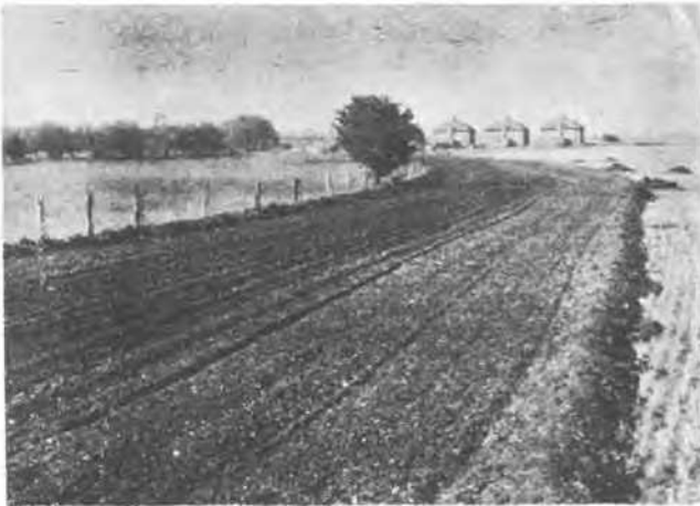
Abingdon:- A view of part of the road during construction.
