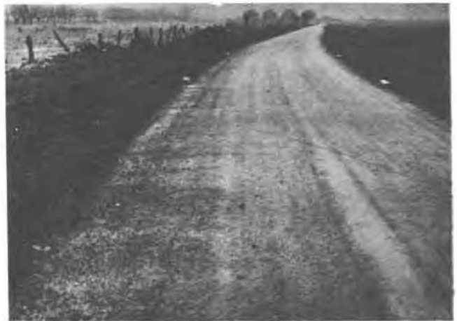
Abingdon:- A view of part of the completed road.
