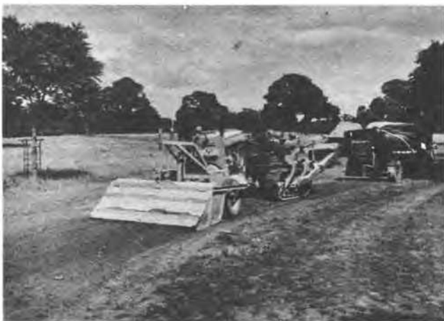
Hatchlands:- Work in progress.
