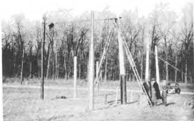
Loading equipment on post 3 Plate 1
