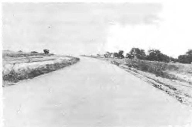
All curves were built with proper super elevation
