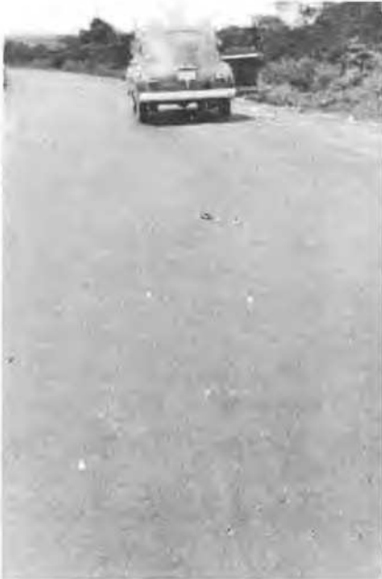
Slight cracking observed near top of some small hills
