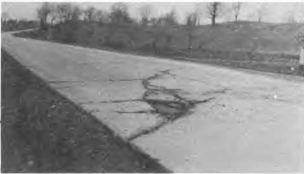
Figs. 11 & 12 Illustrations of maintenance problems which require a subgrade investigation for their proper solution.
