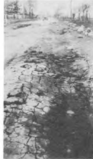
Figs. 11 & 12 Illustrations of maintenance problems which require a subgrade investigation for their proper solution.
