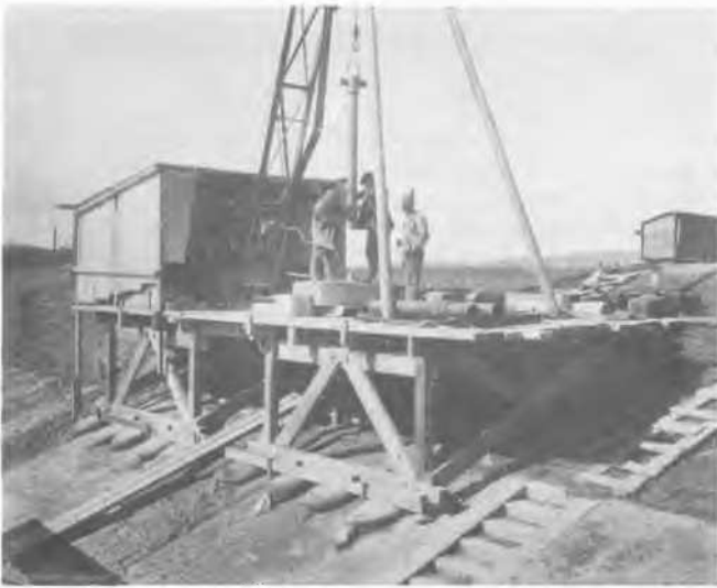
Fig. 3 Setting up a drive pipe (Shannon River)
