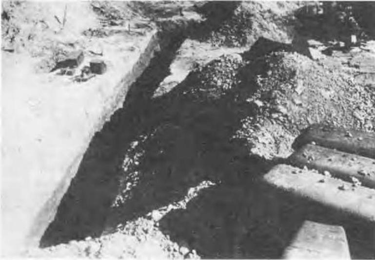
One of the measures sometimes adopted for the protection of structures from vibration is the digging of trenches, sheet piling, or some other barriers, are set up between the structure and the source of vibration. Sometimes these methods are effective, but often they are ineffective; as in their construction the necessary conditions for effectively screening the structure from the above waves are not carried out properly.
