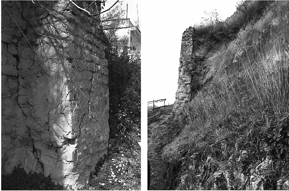
Fig. 9. Examples of deterioration of the system of retaining structures; left: detachment and fracturing of a counterfort; right: collapse of a retaining wall
