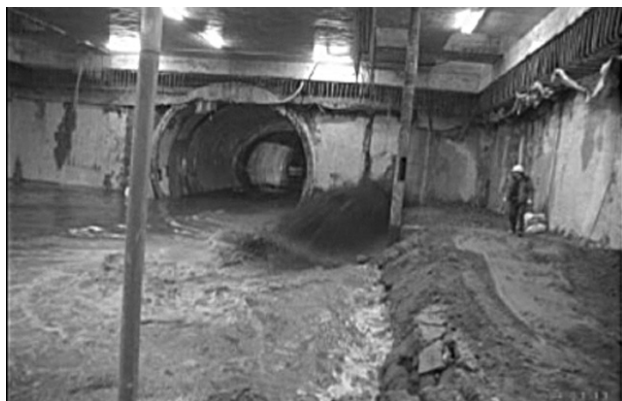
Fig. 31. The inrush of water and sand into the excavation
