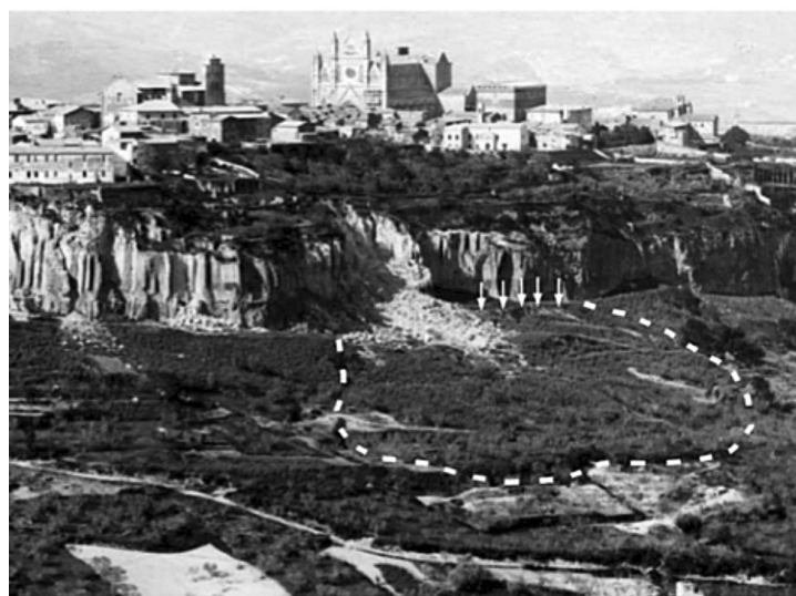
Fig. 18. Orvieto; the collapse of a sector of the tuff slab in 1898. The arrows and the dashed line indicate respectively the crown scarp and the body of the previous landslide on the clay slope.
