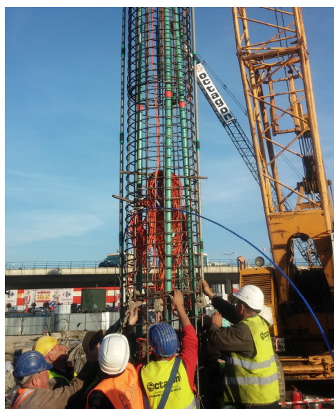
Figure 1. Picture during the installation of the instrumented piles
