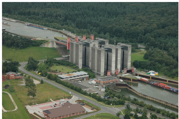
Figure 1. Aerial photograph, north-east view, of the existing Lueneburg twin ship lift.
