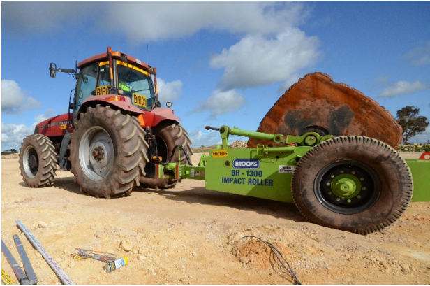
Figure 1. Broons 4-sided, 8-tonne, BH-1300 impact roller.
