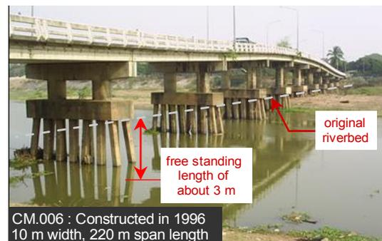
Figure 3. An example case of undamaged bridge which has potential risk of damaging.
