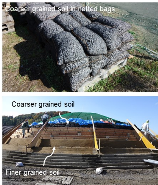
Figure 8. The construction of the double-layered earth mound (September, 2014).
