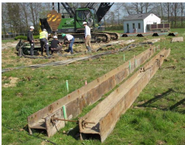
Figure 5. Steel guide used during the vibrodriving phase of the test campaign to guide the sheet piles into the ground
