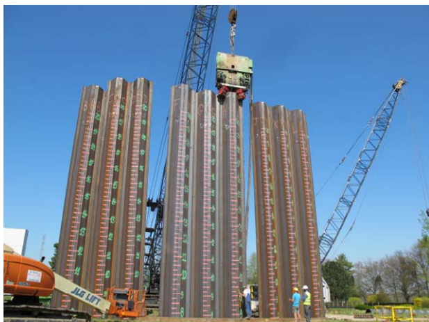
Figure 6. Vibrodriving of the last double sheet pile with the vibrator type Dieseko PVE 40VM on the site of the BBRI
