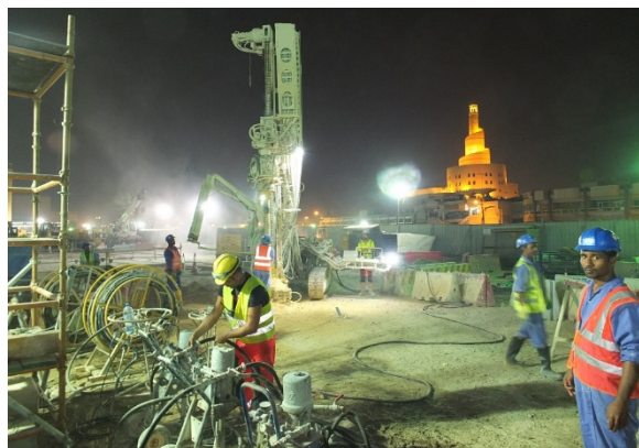
Figure 5. Grouting at night shift
