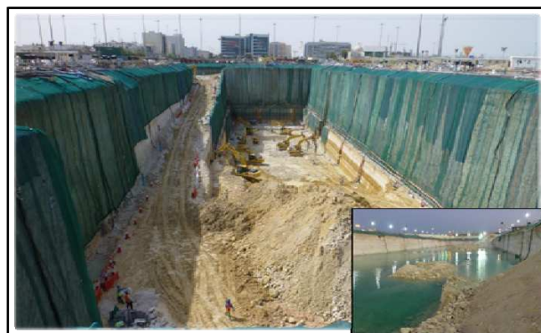
Figure 7. Excavation works pre and post grouting excavation box.
