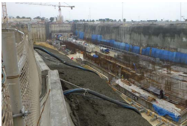
Figure 4. Open cut excavation with grout curtain
