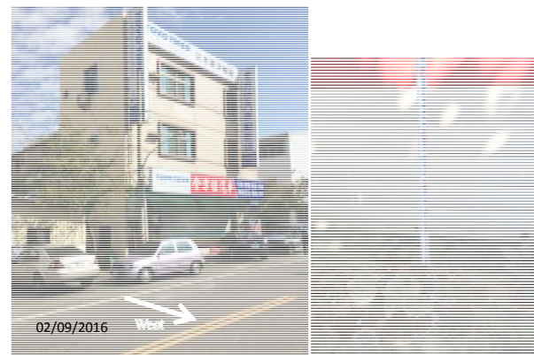
Figure 5(a) and (b) The car repair center faces to the west side with an individual shallow foundation at Locality 3 settled 20 cm and slightly tilted to the west.
