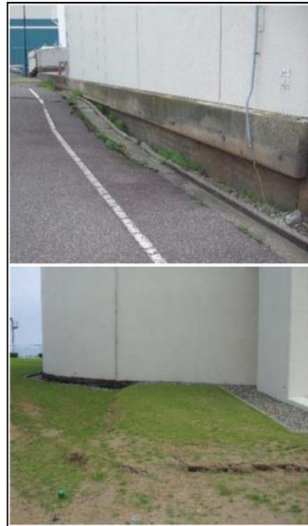
Figure 1. Example evidence of settlement around nuclear power plant infrastructure (taken and modified from Sakai et al. 2009).
