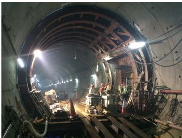
Figure 5. 'Full-moon' support frame in Express Rail Link Tunnel in Hong Kong.
