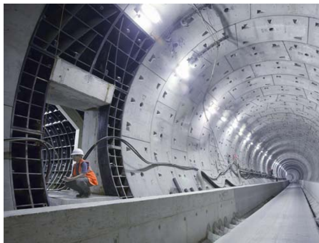
Figure 6. Prefabricated steel segments in Channel Tunnel in the UK.
